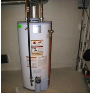
Water Line is Copper Pipe (Upper Right)
