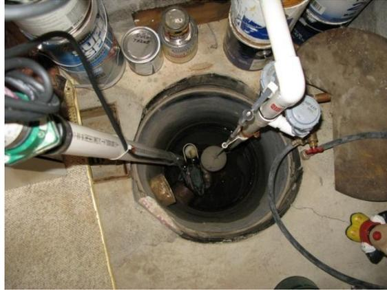
There are 2 types of sump pumps. One type sits on the floor and the other type is mounted in the hole itself.
